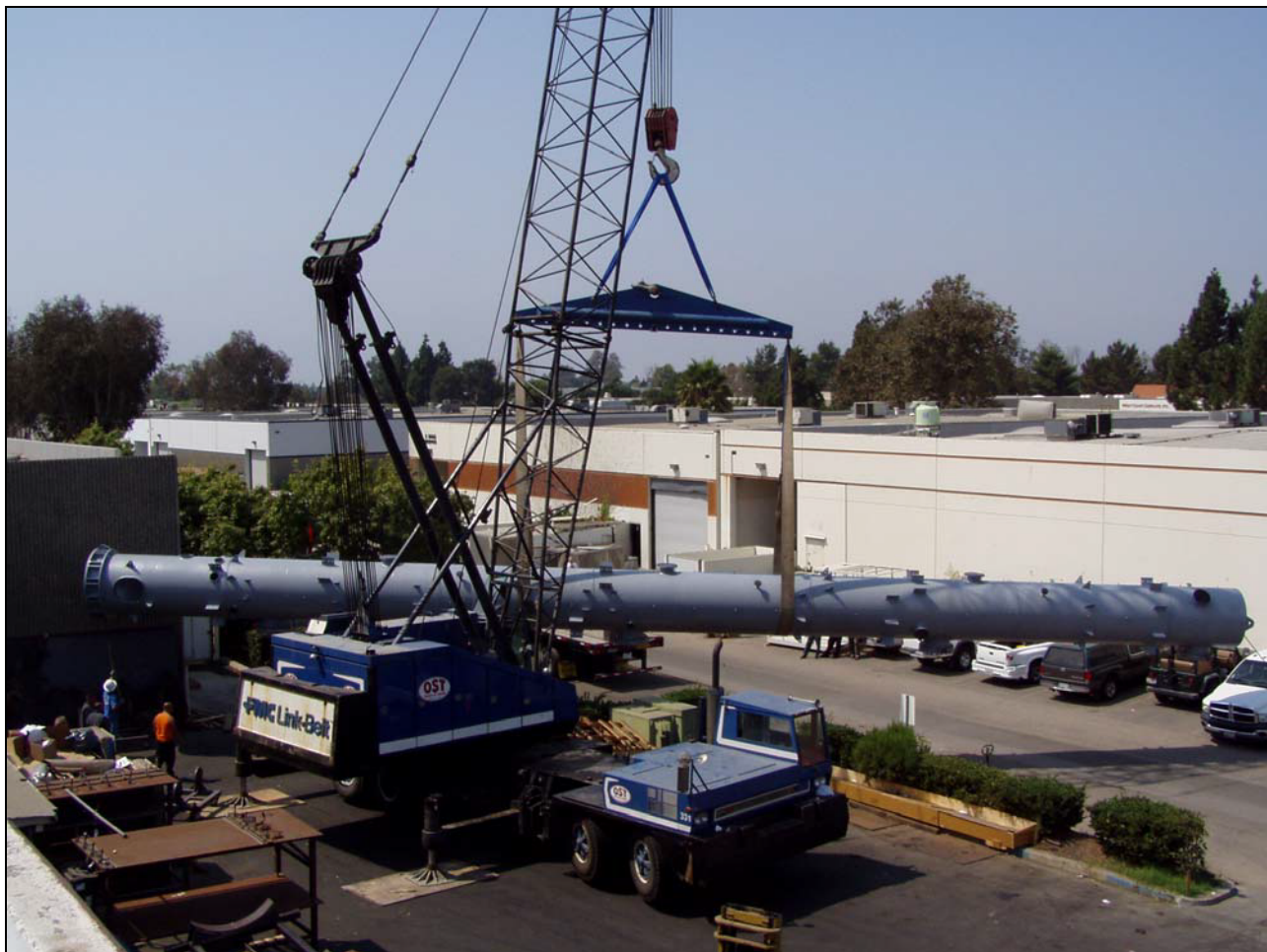
56" DIAMETER X 80 FOOT TALL TANTALUM LINED CARBON STEEL COLUMN
